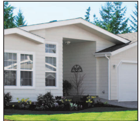
The custom-designed homes at Azalea Gardens come in eight different styles and floor plans. All plans are one-story ramblers with a concrete ramp entry for safety.
